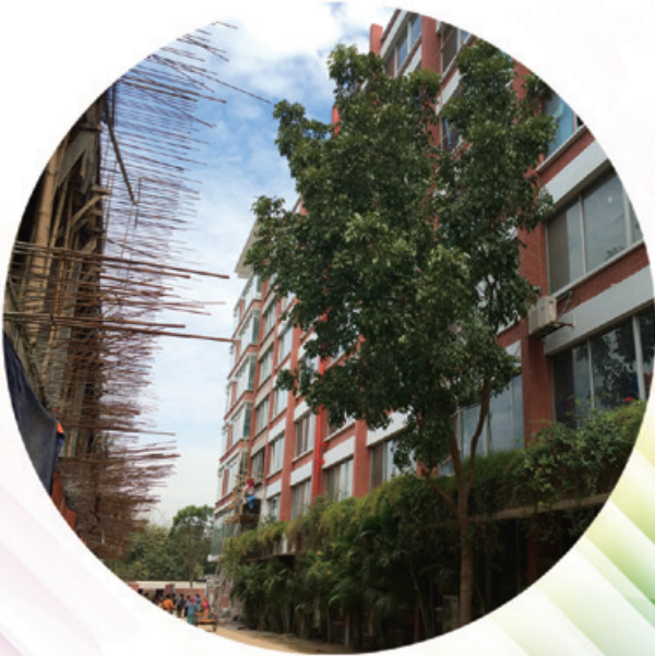
Unimas expansion project is in full swing
